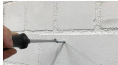
Place the dowels in the holes and fasten the hooks. They should protrude approx. 20 mm.
