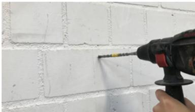
Drill holes using 8 mm drill bit. Drill approx. 45 mm deep.
