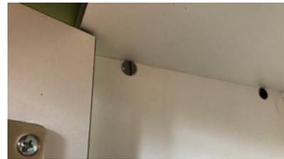
Place the threaded sleeves in the holes inside the Bottom Module. Align the slot vertically.
